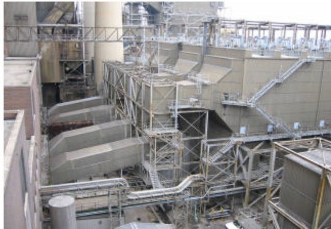
Figure 11. Ductwork leading to the St. Clair ESPs.
